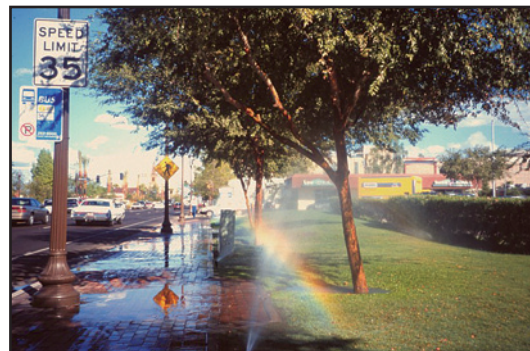
Sprinklers out of adjustment and wind drift
