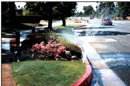
Broken sprinkler floods street and hardscape causing damage
