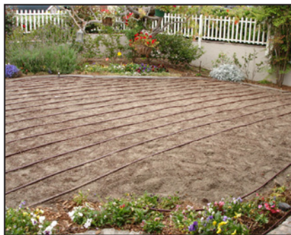
Techline CV dripline turfgrass subsurface installation
