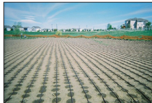
Wetting pattern of Techline CV dripline prior to turfgrass subsurface installation
