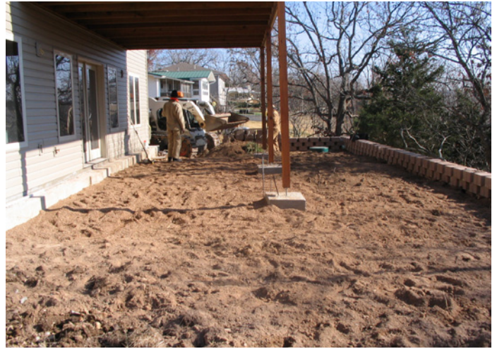
Clean fill is added before dripperline is laid out.
