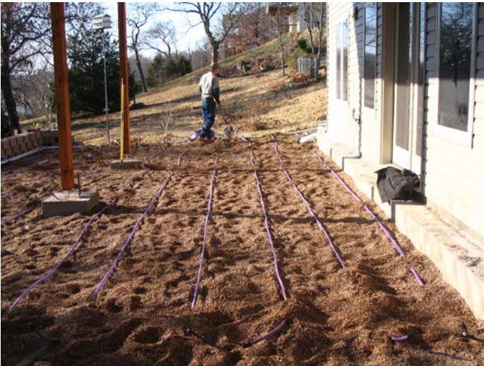
Bioline dripperline is laid out. Note the proximity of the tubing to the home. Bioline's precise application allows it to be used where other products cannot perform, including close to hardscapes.
