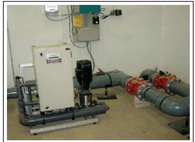
Figure 6. A Netafim fertilizer injection and irrigation control system. Flow meters are located on the right a pressure gauge is visible on the left.
