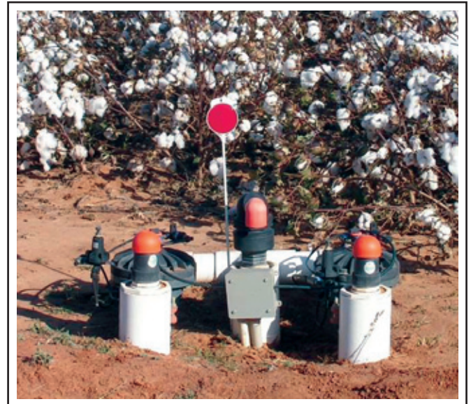
Figure 4. Top photo and photo above are examples of field installation of pressure regulating air and release valves.
