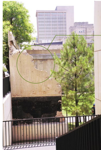
Framing the eastern edge of the field of chairs is the only remaining wall of the Murrah building, a large chunk of ragged concrete and protruding rebar.
