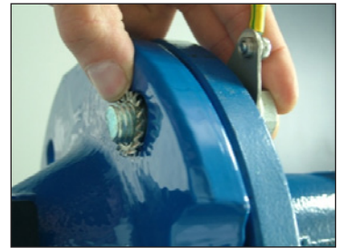
STEP 7 Add serrated washer to the other side of the bolt (on meter's flange side).
